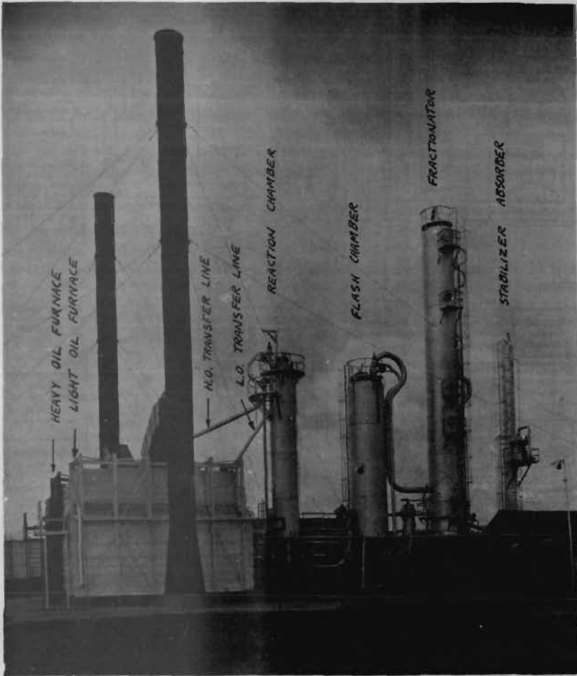
FIG. 14. Universal Oil Products two-coil selective cracking unit.
