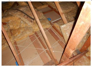
The interior walls of the living room vaulted ceiling have insulation that has fallen out of place (See image below). We recommend replacing the loose insulation and resecuring it to the wall for improved energy efficiency of the home.
