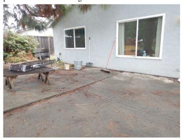
The grade of the soil at the right side of the home encourages storm water to drain toward the structure. Moisture saturation around the foundation could impact the stability of the foundation over time and encourage moisture to enter the garage. The grade should be modified to promote the flow of storm water away from the structure;
