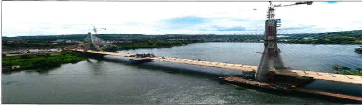
Figure 1: 2nd Nile Bridge, Jinja
