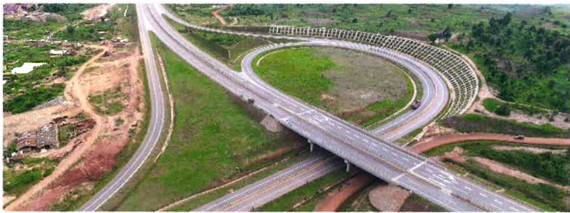
Figure 2: A section of the Entebbe Express Highway
