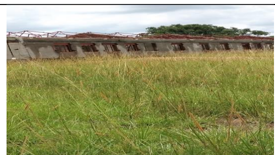
On -going works on ICT & science block
