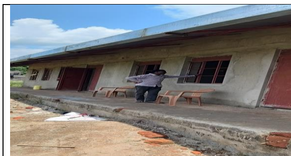
On-going works on administration block
