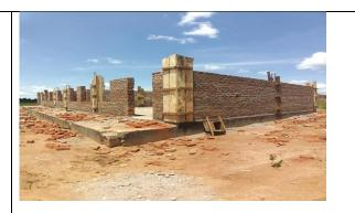
2 unit Science Laboratory block Brick works has reached ring beam level and await casting the columns and beams as well
