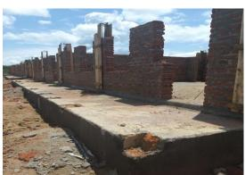
3 classroom Blocks @ 2 class rooms Brickworks has reached beam level and column bars installed and awaits casting the columns and ring beam
