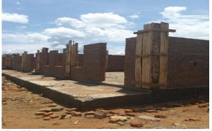
First block of 2 classrooms Brickworks has reached beam level and column bars installed and awaits casting the columns and ring beam
