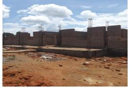
**ICT Block** Column bars installed awaits casting
