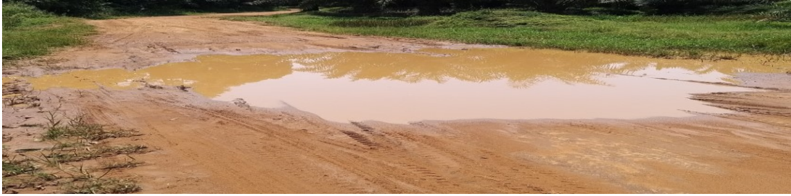
The Road Section that required culverts to make it easily passable.
